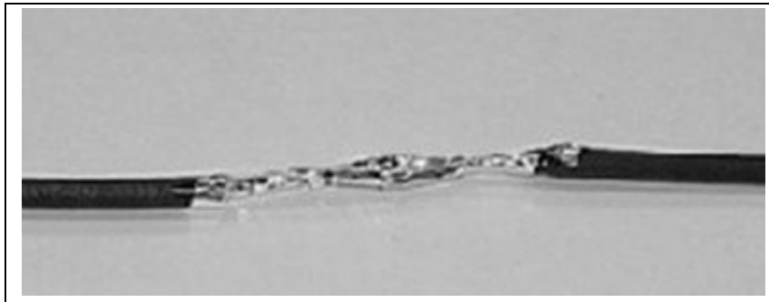
Center Heat Shrink Tube Over Cable
